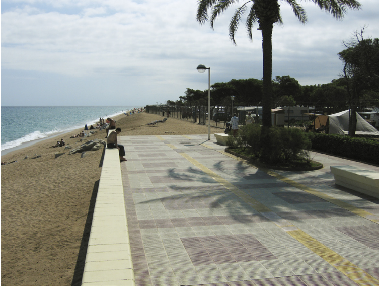
Figure 3. Photographs of the same place on the S'Abanell beach in 2016 and 2017. In 2006, the beach had already been considerably reduced in area due to the decrease in fluvial inputs and marine storms. In 2017 the beach has completely disappeared and it was necessary to build a breakwater with large blocks of stone to protect a campsite and prevent the displacement of people. Source: Pictures by the author (8/2016 and 1/2017).
