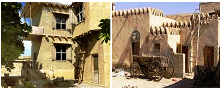
Figure 2. Traditional rural houses in Egypt: house of red bricks and house of mud bricks. Source: Eisa (2014: 186).
